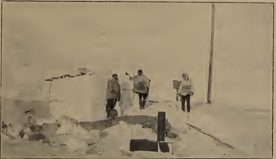
BUILDING THE SNOW WALLS (ON PRINCIPLES ENTIRELY DIFFERENT FROM THE REAL ESKIMO SNOW-HOUSE) FOR THE OUTER HOUSE WITHIN WHICH THE TENTS WERE TO BE PITCHED FOR WINTER.
